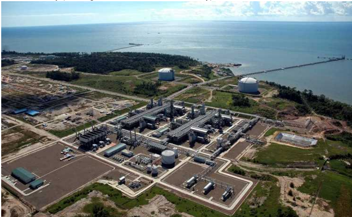
< Plant Facility (existing 2 trains, LNG tanks and Jetty) >
